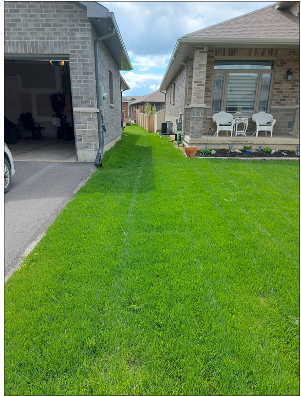
Example of a side yard swale
