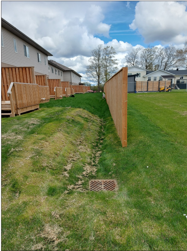
Example of a rear yard swale
