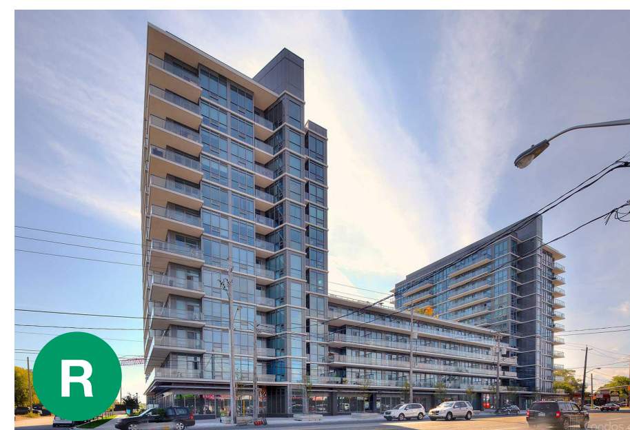
Tower/Podium, Mixed-Use Residential (Toronto, ON)
