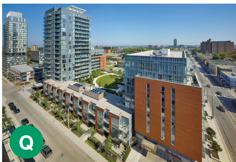
Tower/Podium Mixed-Use Residential (Toronto, ON)
