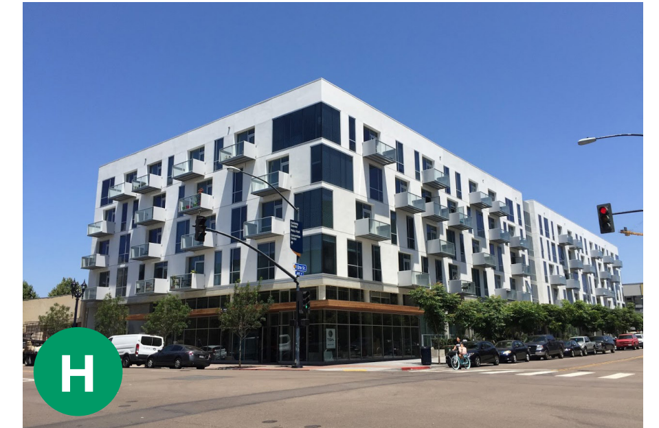
5-storey Mixed-Use Residential (San Diego, CA)
