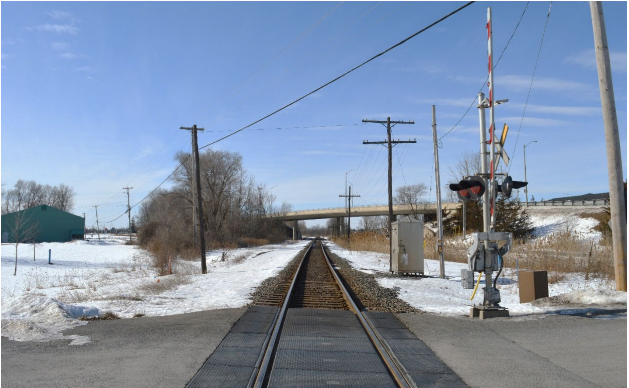
Figure 2: An at-grade crossing of the CP rail line.
