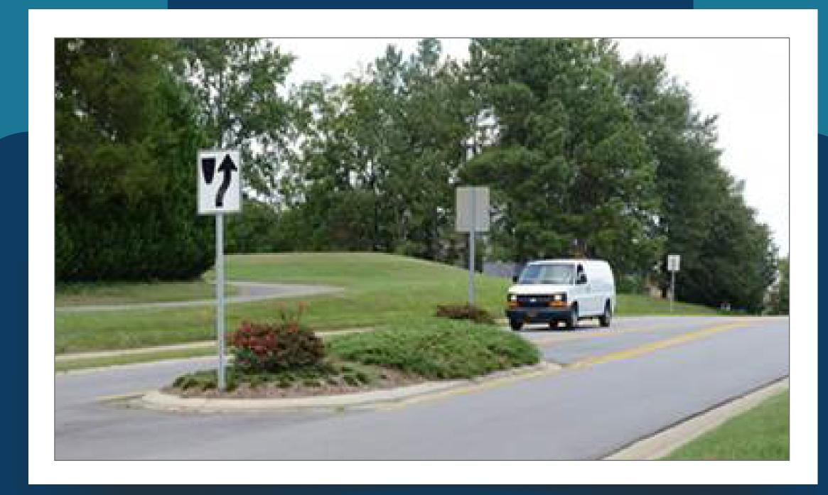
An elevated median constructed on the centerline of a two-way roadway to narrow the roadway.
