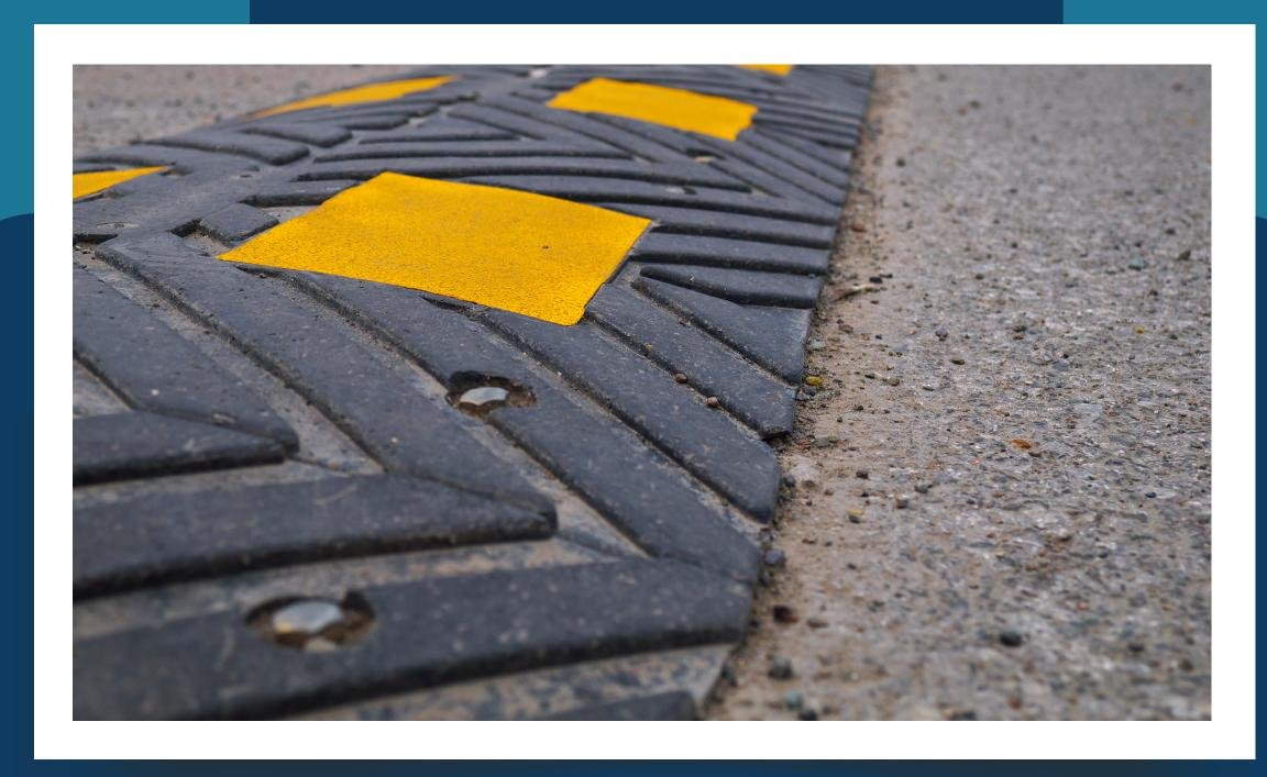
A raised area of a roadway, which deflects both the wheels and frame of a traversing vehicle. Properly designed speed **humps** are not to be confused with speed **bumps**, which are sometimes installed on private roadways and in parking lots and can be very abrupt and jarring to motorists.
