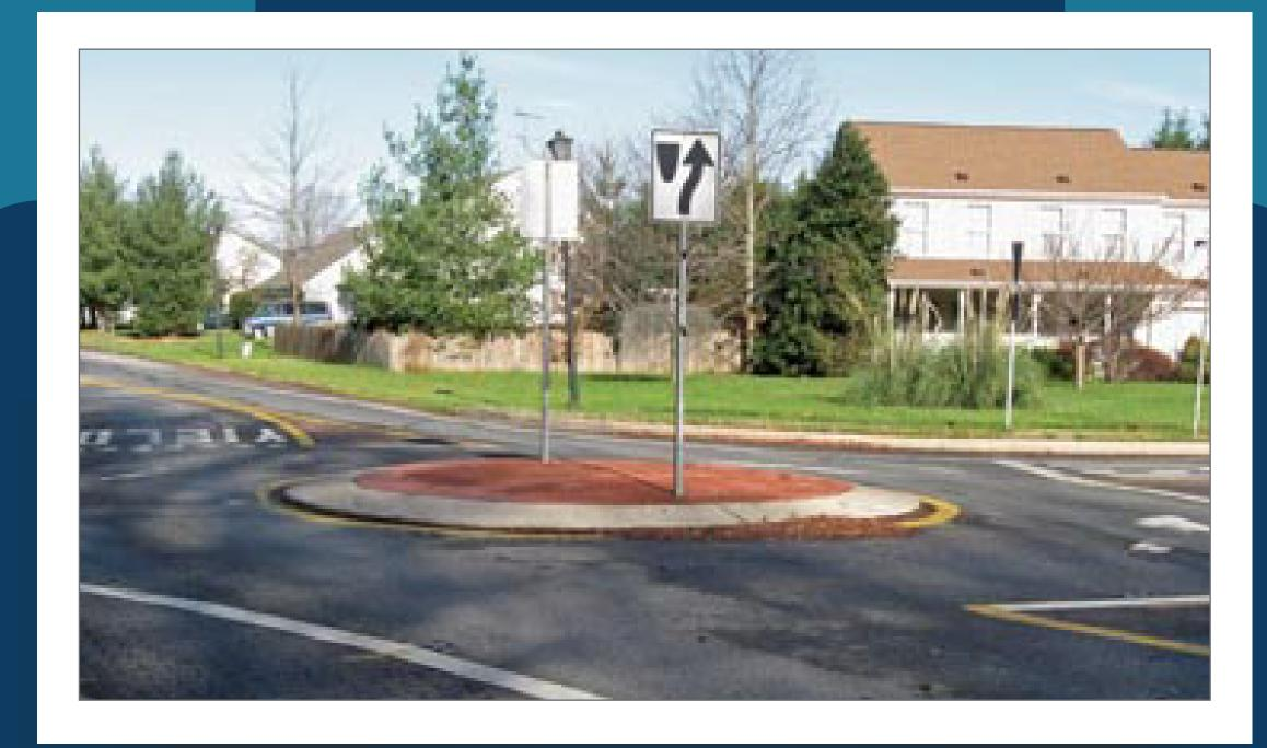
A raised island located in the center of an intersection, which requires vehicles to travel through the intersection in a counter-clockwise direction around the island.
