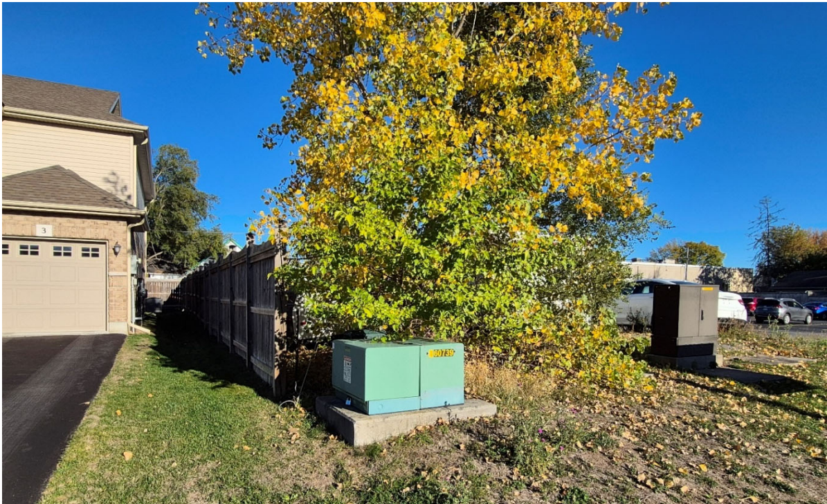
Figure 2: Looking east along northern property line
