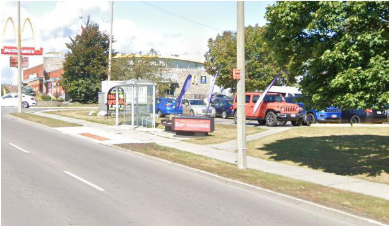
Figure 67: Belleville Transit Bus Stop on North Front Street northbound at Donald Street. This is a near-side stop with a shelter and an appropriately sized pad.
