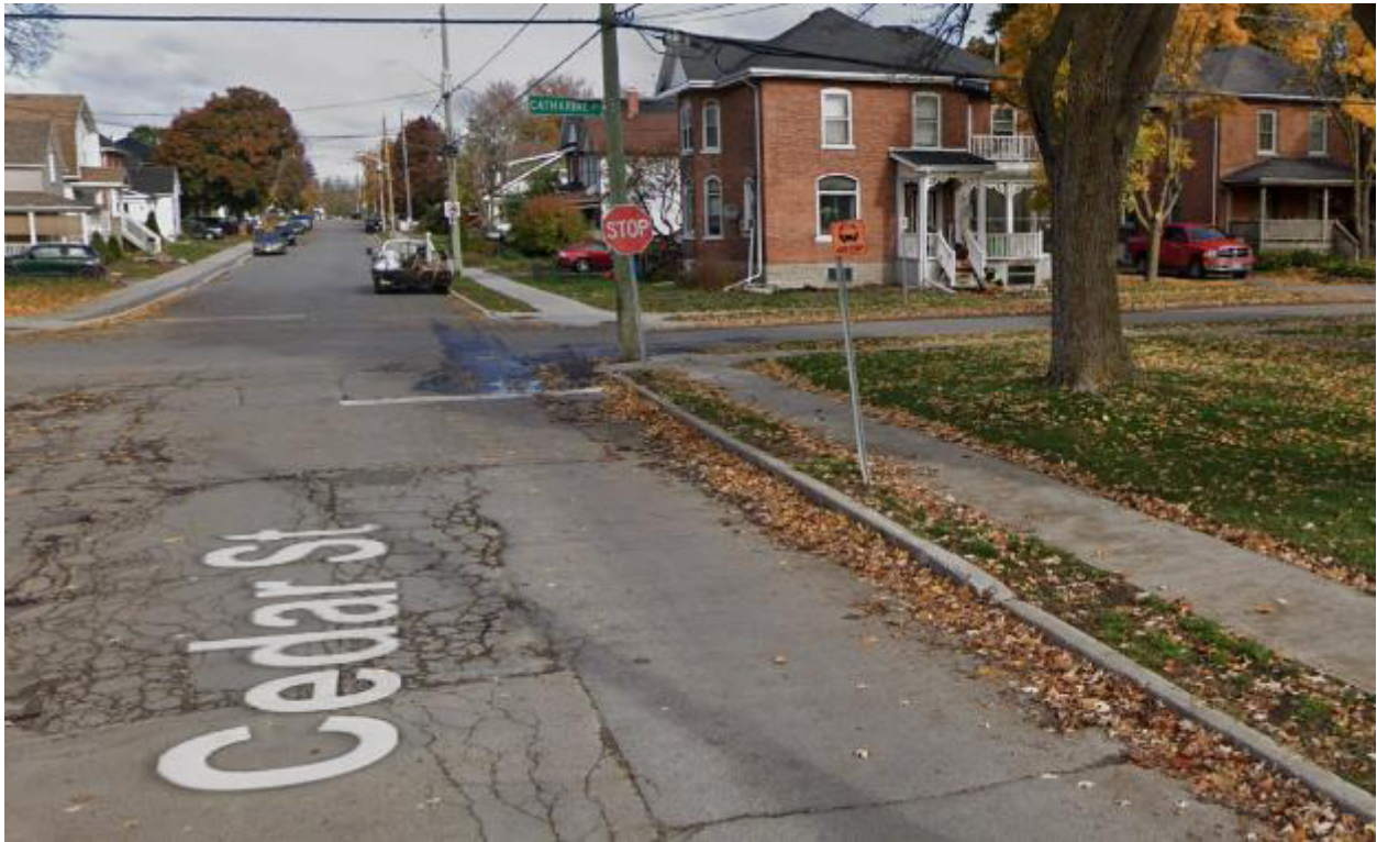
Figure 61: Belleville Transit Bus Stop on Cedar Street at Catherine Street. This is a near-side stop on a neighbourhood street with no pad or shelter. Insufficient space between stop sign and intersection.
